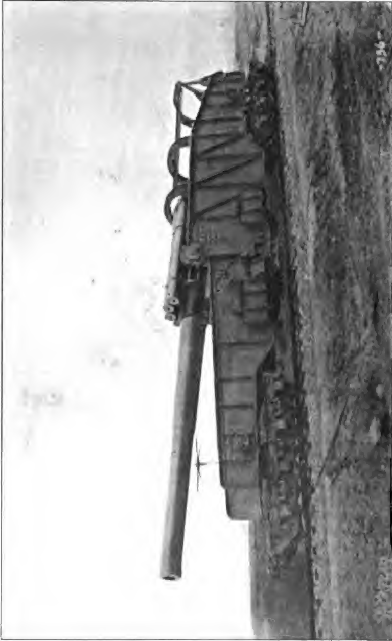
14-INCH, 45-CALIBER AMERICAN GUN ON RAILWAY MOUNT, MODEL "E" (LEFT SIDE).
